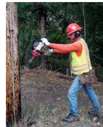
After excavation and inspection, UPT Treating Technician Kristopher Barnes applies a wood preservative paste on a PG&E pole near Hanford, California. In the vast, flat, agricultural terrain of the Central Valley, inspection and treatment work tends to go faster.
