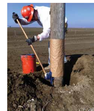
After excavation and inspection, UPT Treating Technician Kristopher Barnes applies a wood preservative paste on a PG&E pole near Hanford, California. In the vast, flat, agricultural terrain of the Central Valley, inspection and treatment work tends to go faster.
